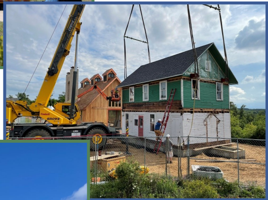
The Brewing Experience Building and Tavern Fall 2021
